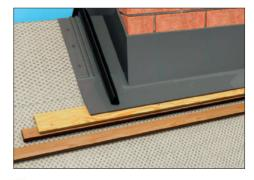
7b A batten and flashing support timber are now fixed in place under the bottom flange of the chimney. This provides support for lead flashing apron. It is important to ensure that this supports the lead sufficiently to prevent ponding.
