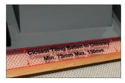
7a Before battens are secured 1No tiling batten must be fixed at front of chimney. This should be installed with a min 75mm to max 150mm below the GRP front edge flange.
