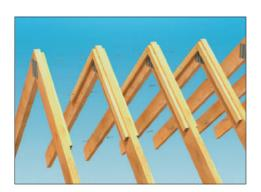
To fix support board, secure 2 No. battens to the inside face of both rafters so both battens are facing each other. Repeat for each rafter space.
