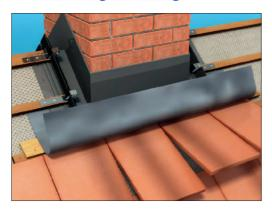
9a Ensure flashing is rolled back to clear working area. Secure extra batten to act as support for ply section. Note batten must extend further than flashing.
