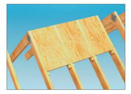
1c Secure the fixing support boards between the rafters with stainless screws at 300mm centres into each batten.
